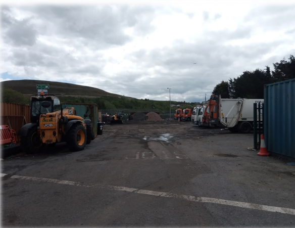
EXISTING CENTRAL DEPOT
